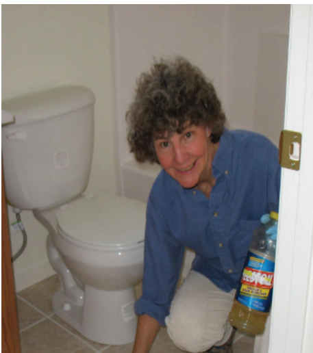
Andrea scrubbing with tooth brush before sealing grout at Fetterly House
