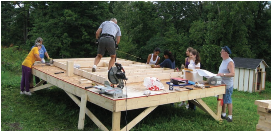
Volunteers Working At Breed Road Site
