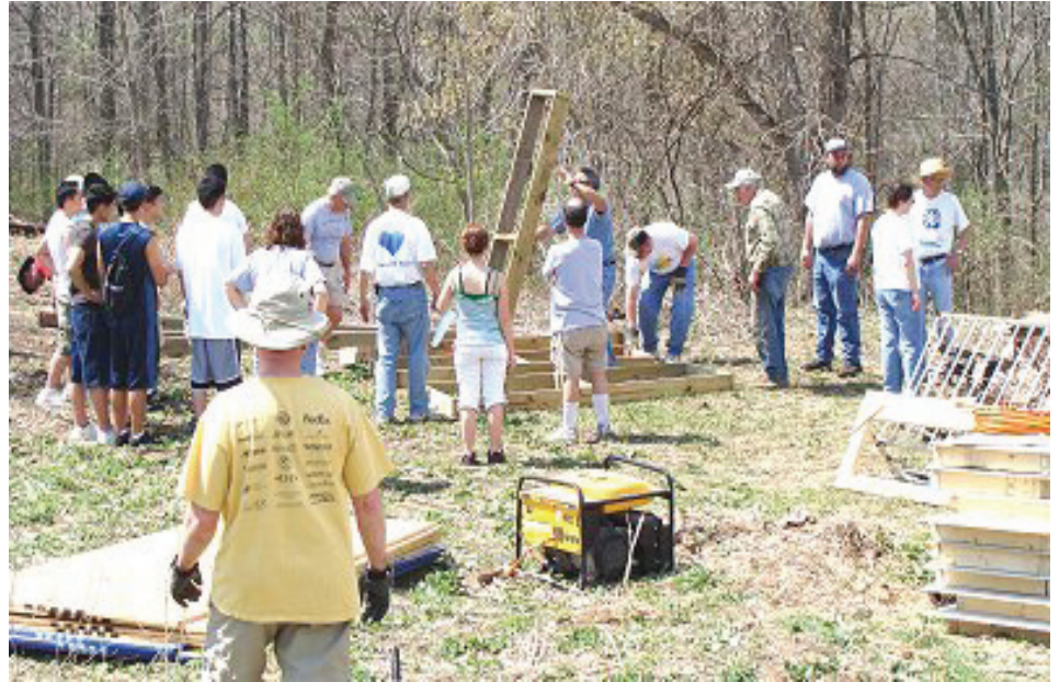
Shed Building at Breed Road
