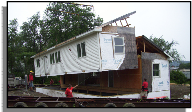
American Homes crew setting the house
